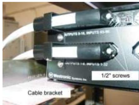
Figure 5 – Typical WS3500 50-pin cable connection
